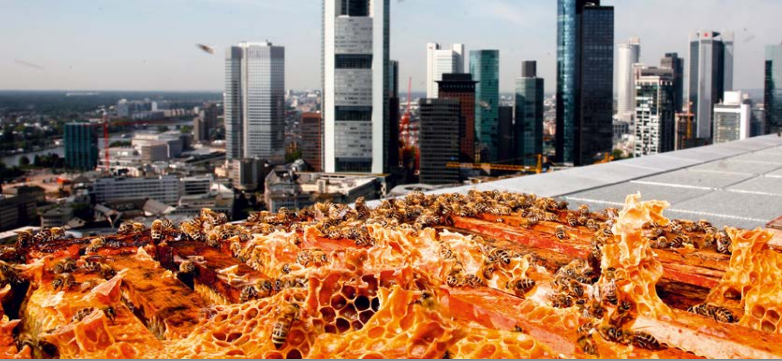
Andreas Wolf keeps bees on the roof of the luxury Jumeirah hotel in the MyZeil Frankfurt building complex, which has been fitted with TROX technology.
