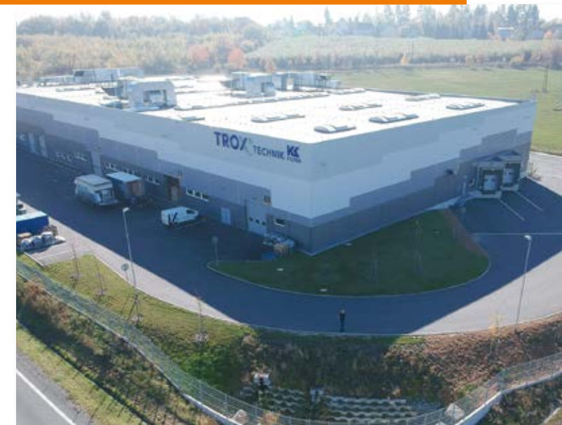
Manufacturing facility of TROX KS Filter.
