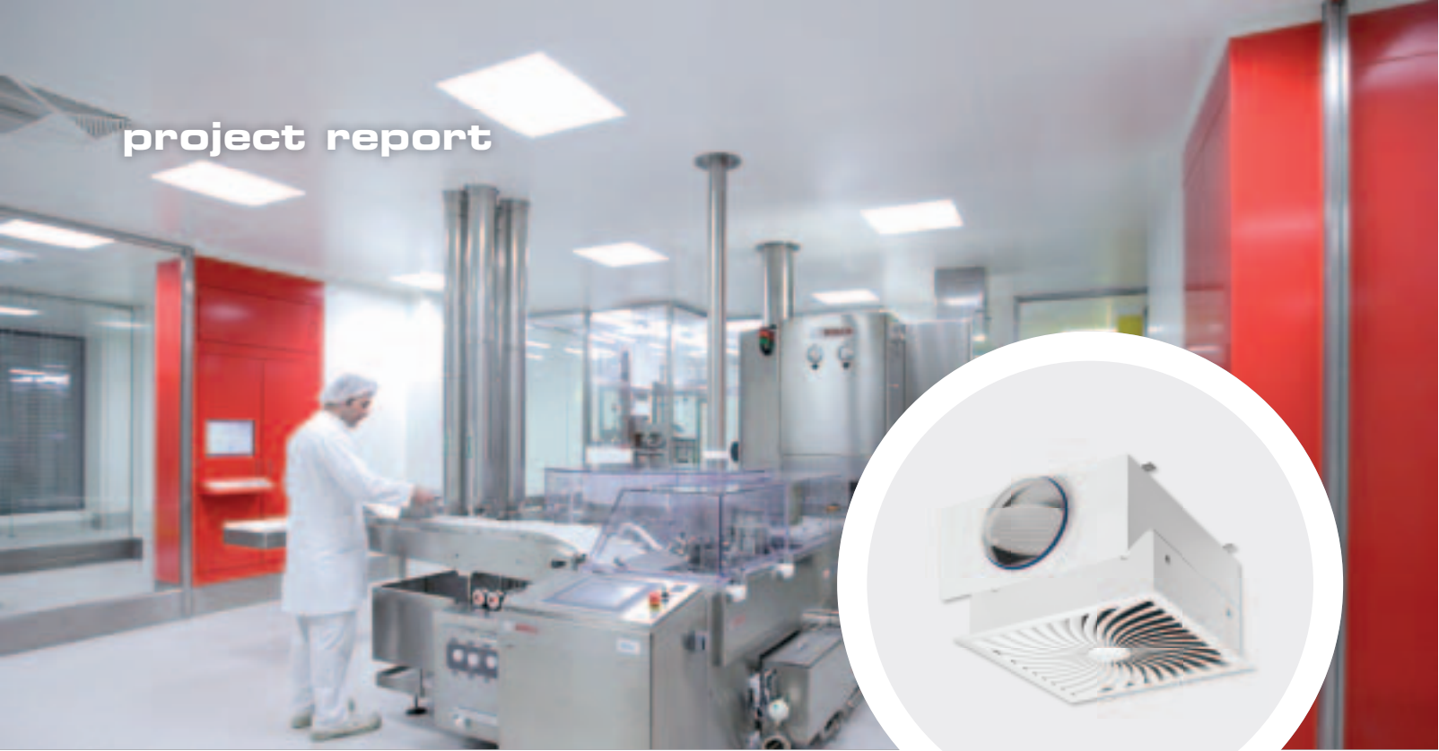
Clean room at the Max Planck Institute, with TROX particulate filter air terminal devices
