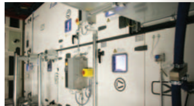
In the clean room test lab in Berlin the TROX X-CUBE air handling unit is used to supply conditioned fresh air.
